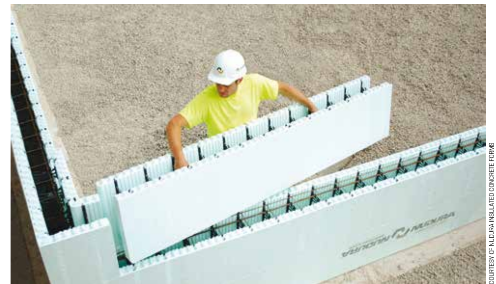
Staying power. NUDURA’s advanced insulating concrete form (ICF) design combines two panels of Expanded Polystyrene (EPS) foam with the structural strength and thermal mass of concrete, for a house hurricane wind resistance up to 250 miles per hour and an energy-efficiency rating as high as R-50.
