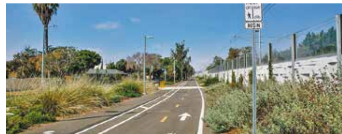
Showing (bio)diversity. The Expo Line Phase 2 project's landscaping design uses native drought-tolerant plant species and recycled water supplemented for irrigation to conserve potable water consumption, reduce stormwater runoff and promote a more natural state of biodiversity.
