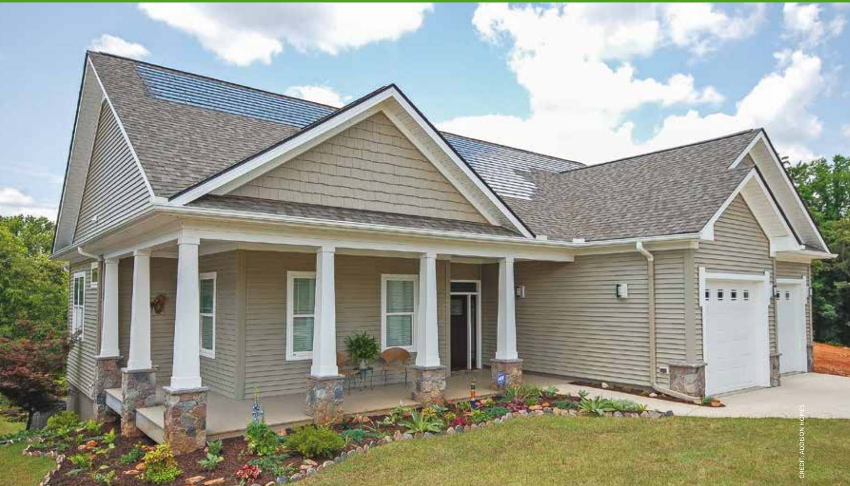
Triple threat. Trailside Community in Greenville, S.C., is Addison Homes' third project to receive a Department of Energy Housing Innovation Award.
