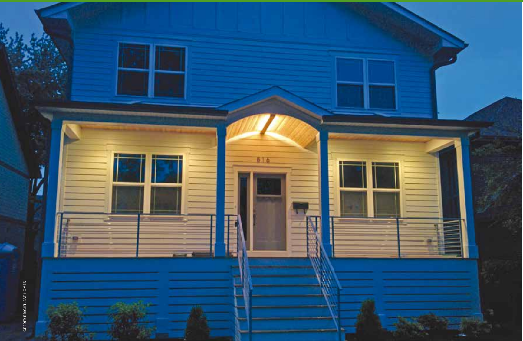
Best face forward. Careful siting of the home optimizes solar gain, and overhangs reduce excess heat in warm months.
