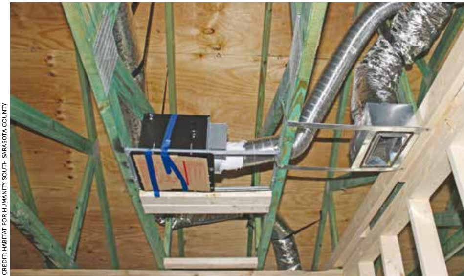
Bug proof. All Habitat for Humanity South Sarasota County homes are built with borate-treated wood framing to discourage termites and other pests from compromising the building structure.
