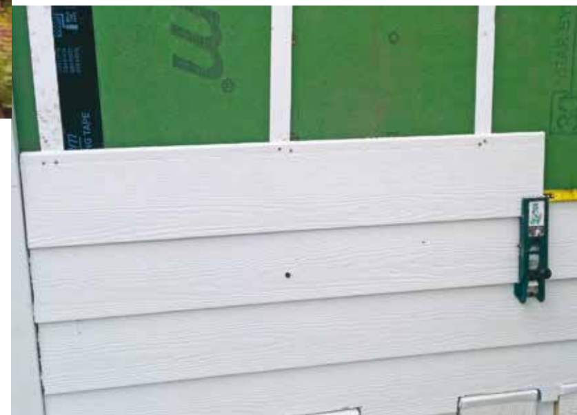
Solid state. The home's exterior is covered with 0.5-inch engineered sheathing with a plastic coating on the exterior side. Similar sheathing on the roof offers an ideal backing for photovoltaic panels.
