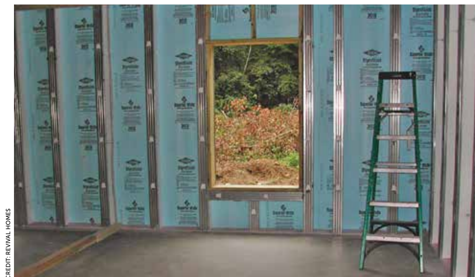
Hard to hole. The home’s first-floor walls are made of precast structural concrete wall panels, consisting of R-12.5 of rigid XPS foam—adhered to a 2.5-inch layer of concrete.
