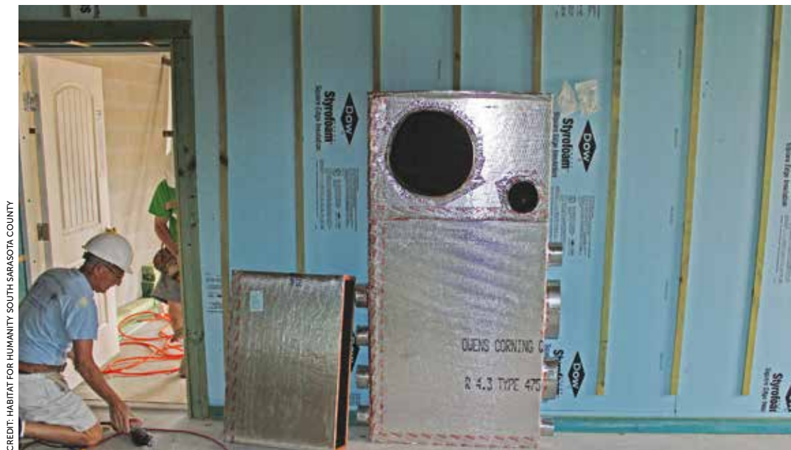
Tough stuff. To increase the insulation value of the walls, hollow cores are filled with a thick layer of rigid expanded polystyrene foam board. In addition, comprehensive air sealing helps keep humidity, pollen and dust out of the home.
