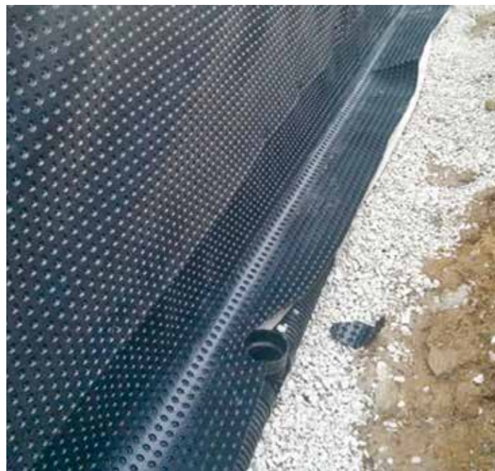
Rain guard. Plastic drain mats protect basement walls from water infiltration.
