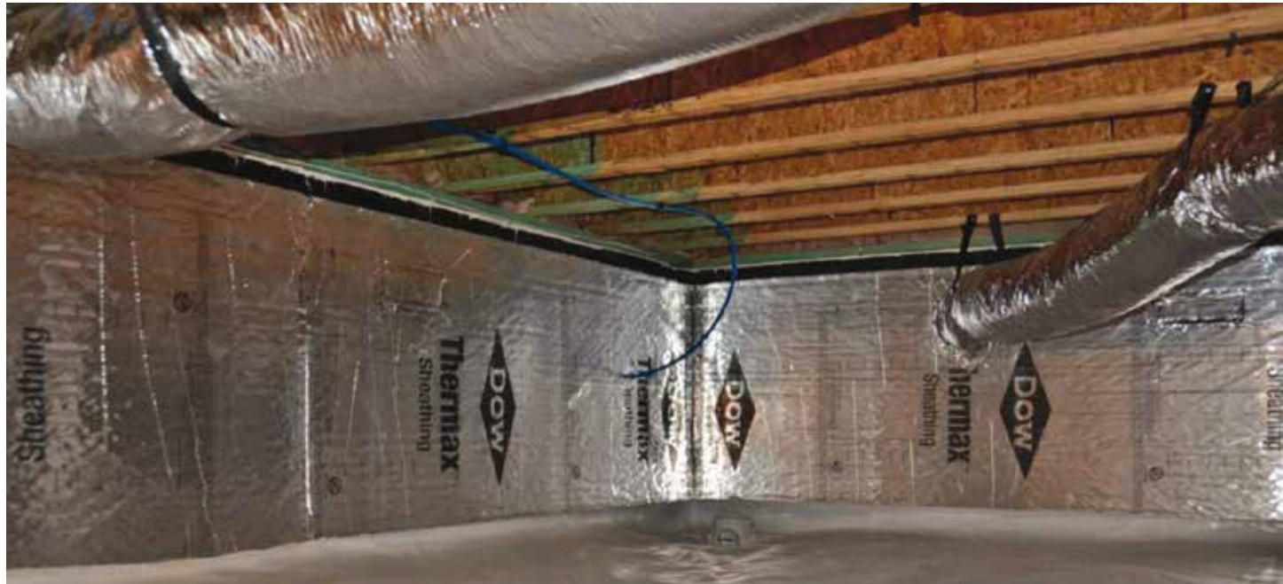
Locked in. Ductwork consists of insulated and air-sealed rigid trunk and flexible branch ducts for improved performance.
