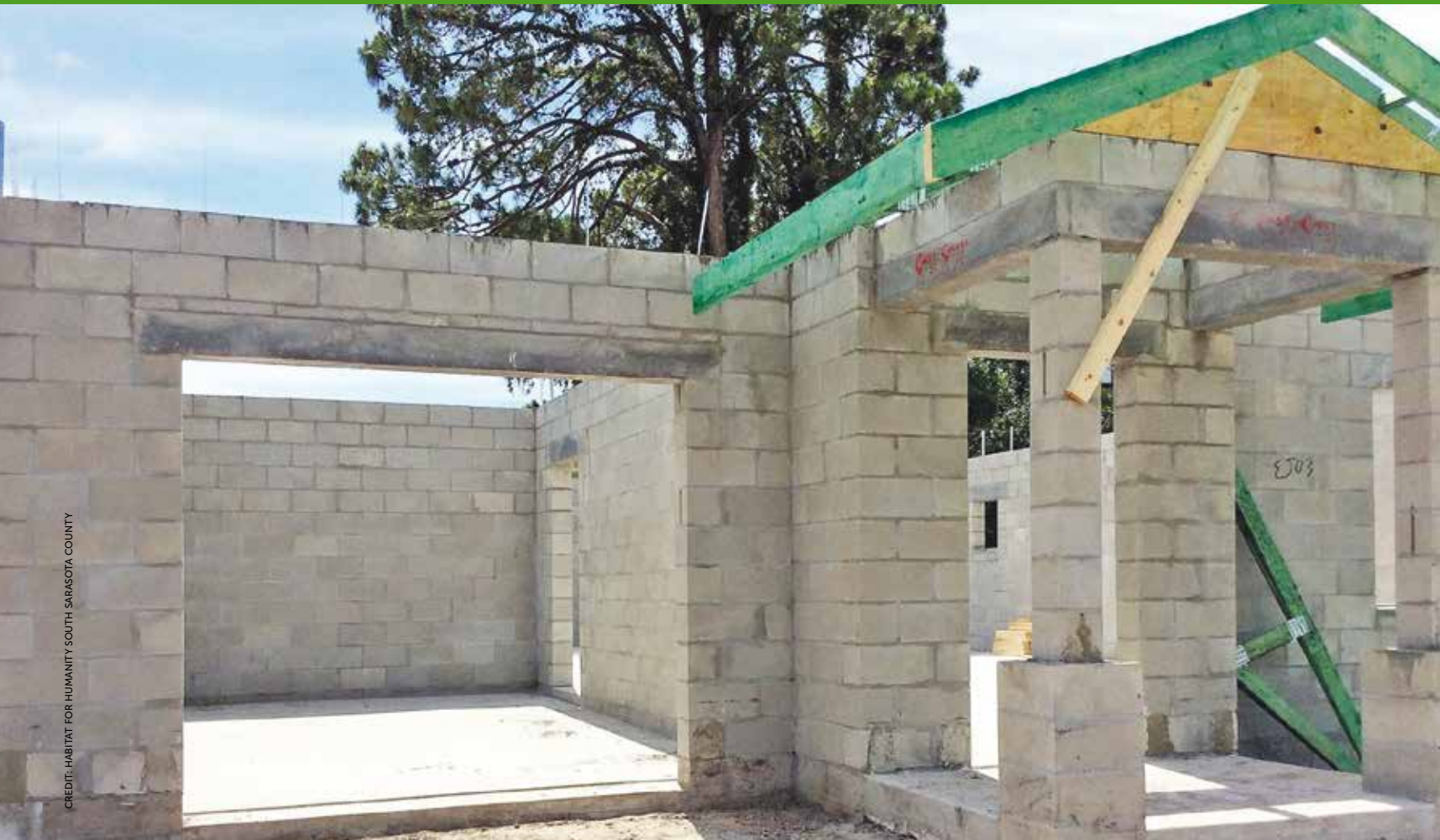
Mass effect. Traditional concrete masonry block walls and a stucco exterior moderate the home temperature fluctuations.
