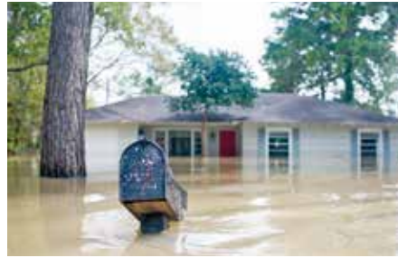
Washout. Recent hurricanes have caused millions of dollars in property damage in cities like Houston, leading to constant rebuilding of homes and other structures.
