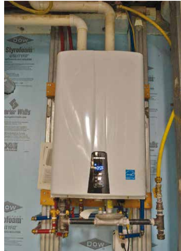
Smart plumbing. Now-standard power-saving devices include an Energy Star-labeled tankless condensing gas water heater with low NOx emissions and a smart controller that learns occupants' hot water usage patterns and circulates hot water when the residents are most likely to need it.
