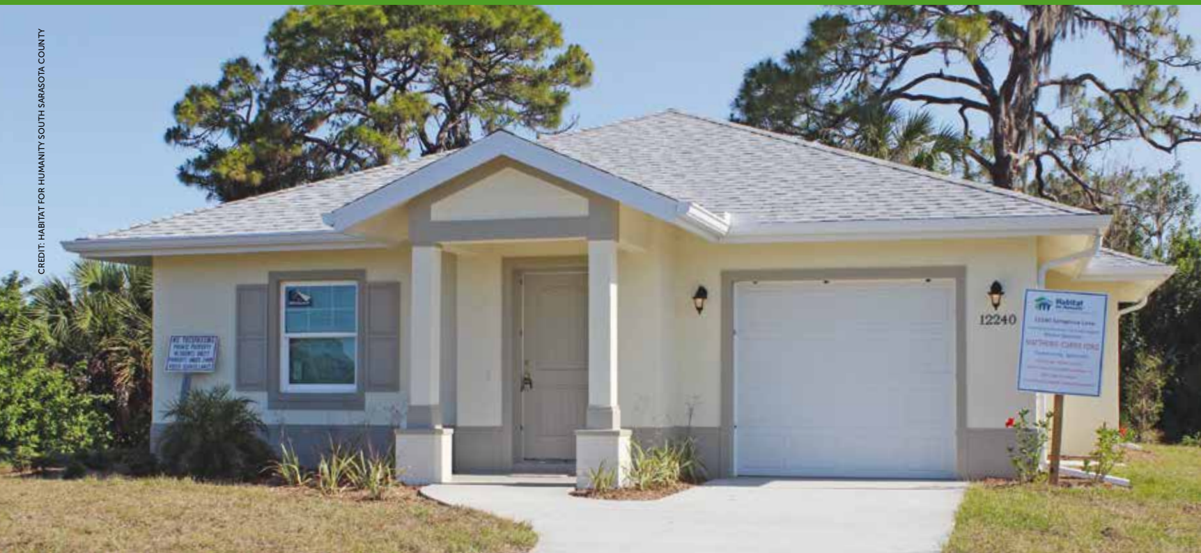
Simple science. Habitat for Humanity of South Sarasota County constructed a modest, energy-efficient 1,200-square-foot home tailored to moderate-income families that is attractive, durable and affordable.
