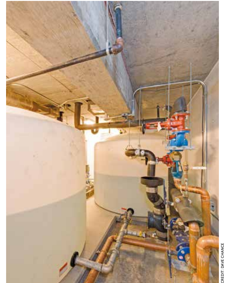
All right as rain. Rain cisterns at Chesapeake Bay Foundation's Brock Environmental Center capture water that is then treated for all potable uses. It is the only building thus far approved by governing health officials for drinking.
