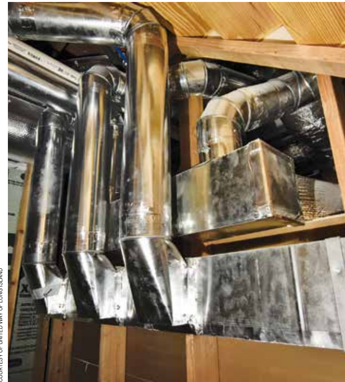
Air force. An elaborate ERV works in conjunction with the home's boiler, fan coil and AC to provide whole-house ventilation and humidity control.
