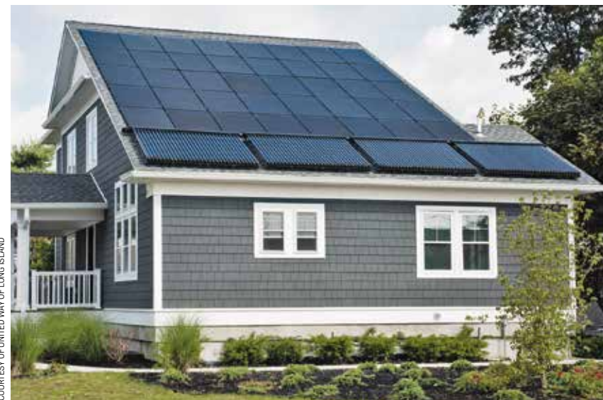
On the slanted side. Beacon House's asymmetrical, optimally angled roof provides plenty of space for roof-mounted solar panels for electric generation and hot water.
