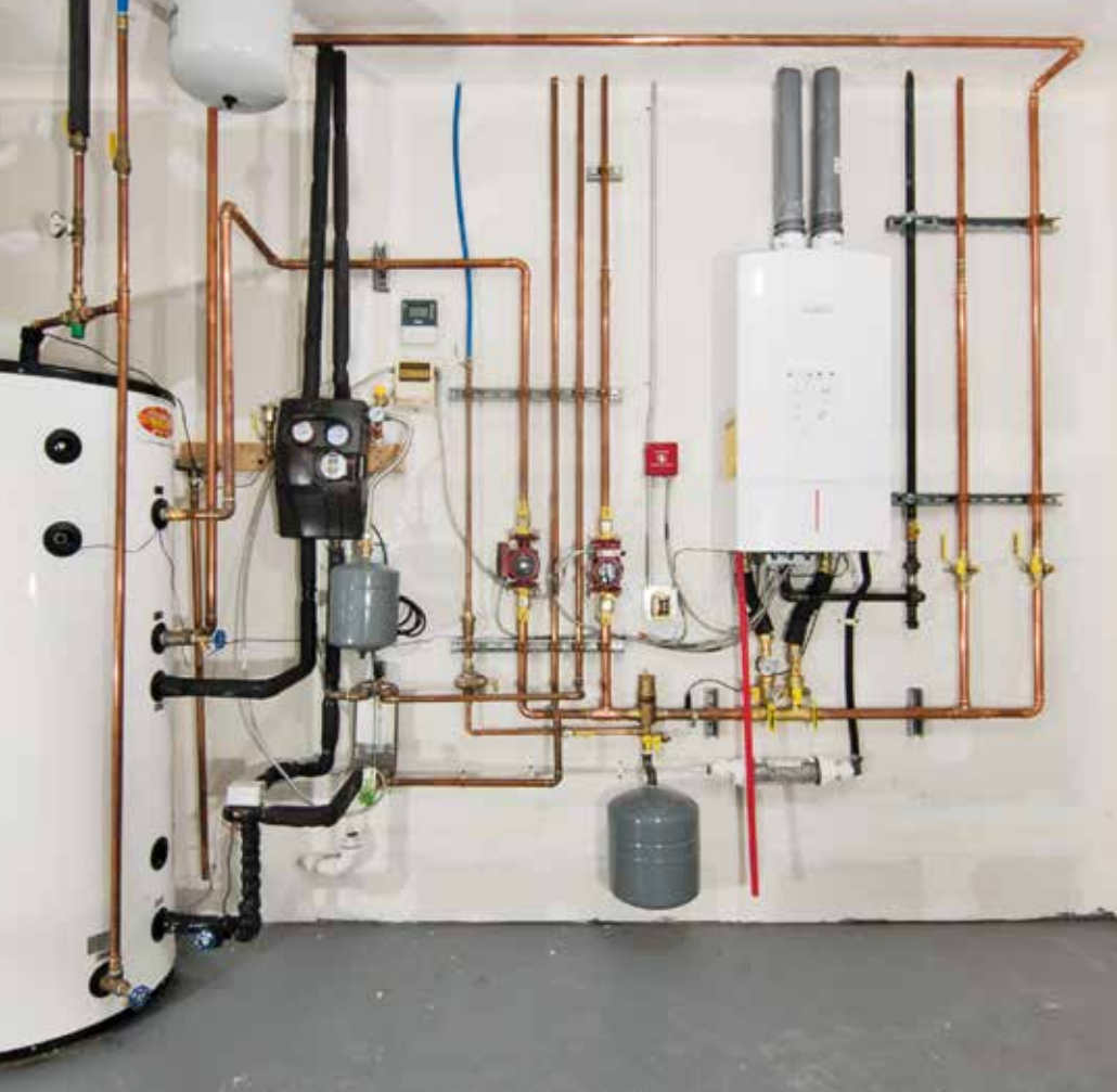
Pipe dreams. A wall-hung boiler feeds a super-insulated, 120-gallon storage tank that can meet up to 85 percent of the home's hot water needs.
