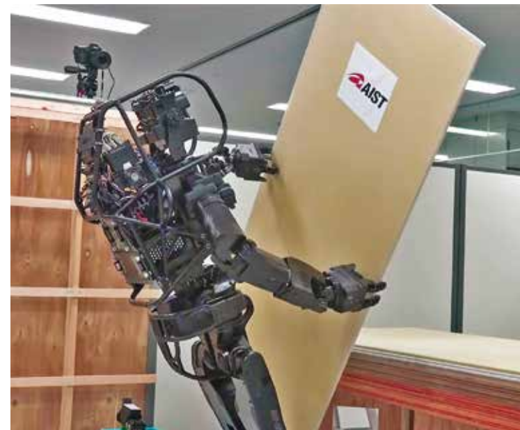
Automated effort. Japanese public research body, National Institute of Advanced Industrial Science and Technology (AIST) is developing a robot capable of activities such as drywall application and wall panel installation. CREDIT: AIST
