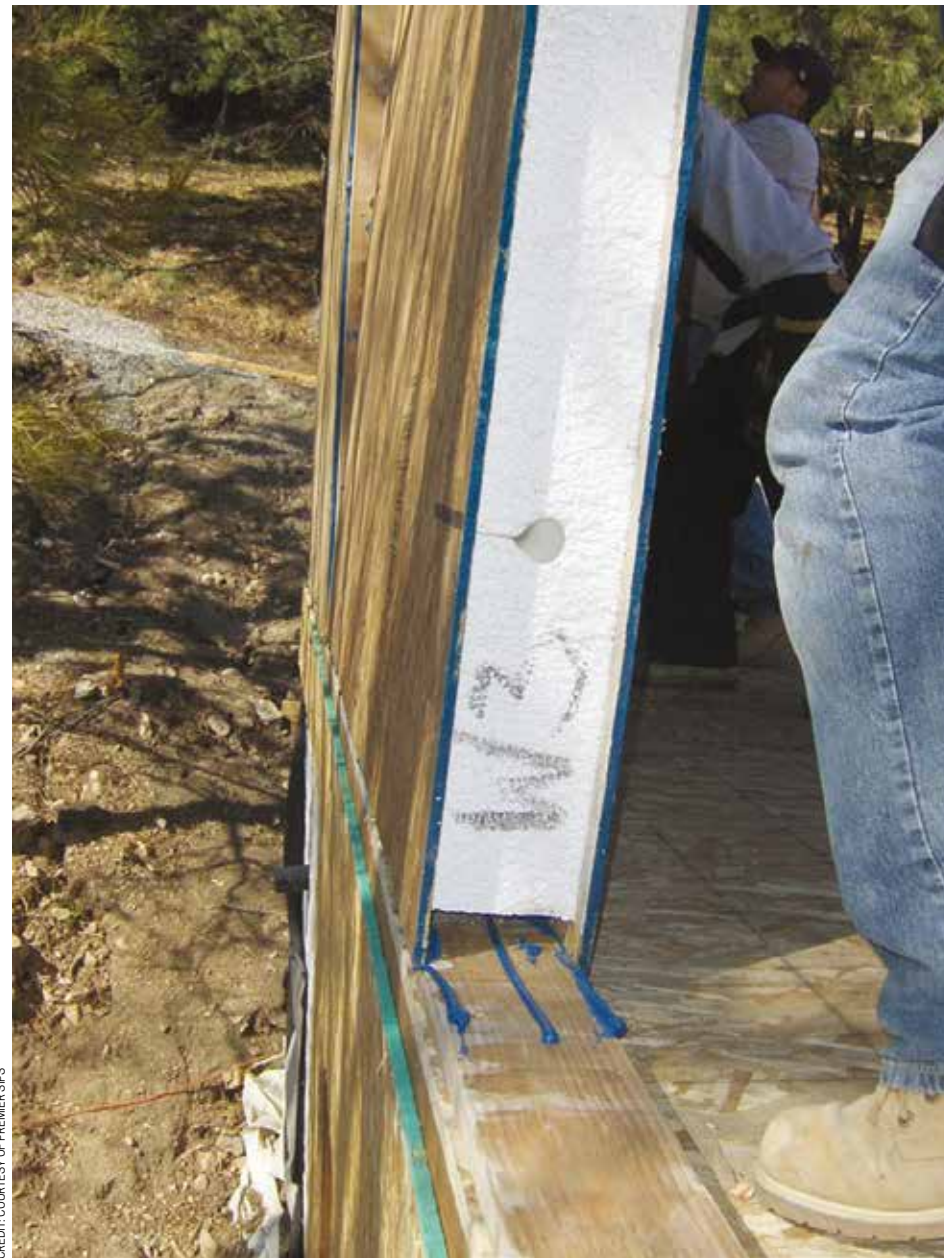
Electric ready. Precut chase cavities in this Premier SIP will save electricians from drilling hundreds of holes through stud framing.
