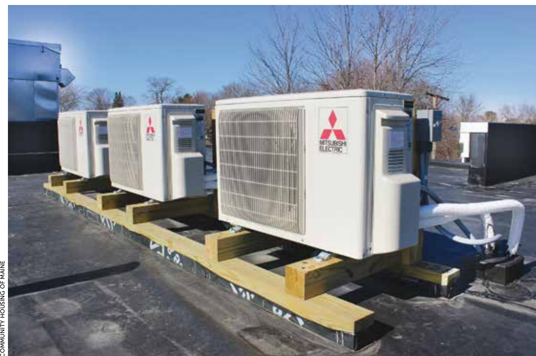
Power play. Photovoltaic panels and rooftop HVAC units helping make Village Centre Apartments 60 percent more energy efficient than a typical code building.
