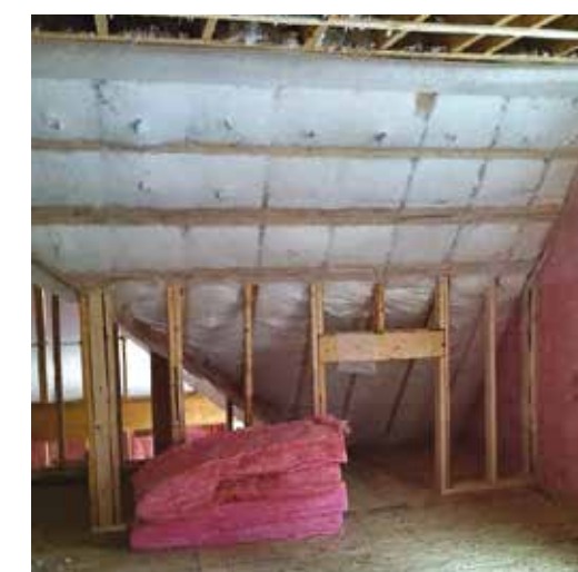
Vented Roof Slope Assembly
