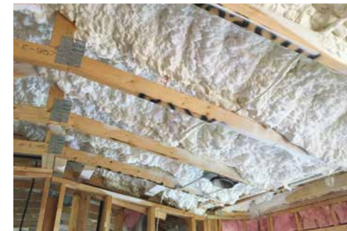
Spray Foam Roof Assembly
