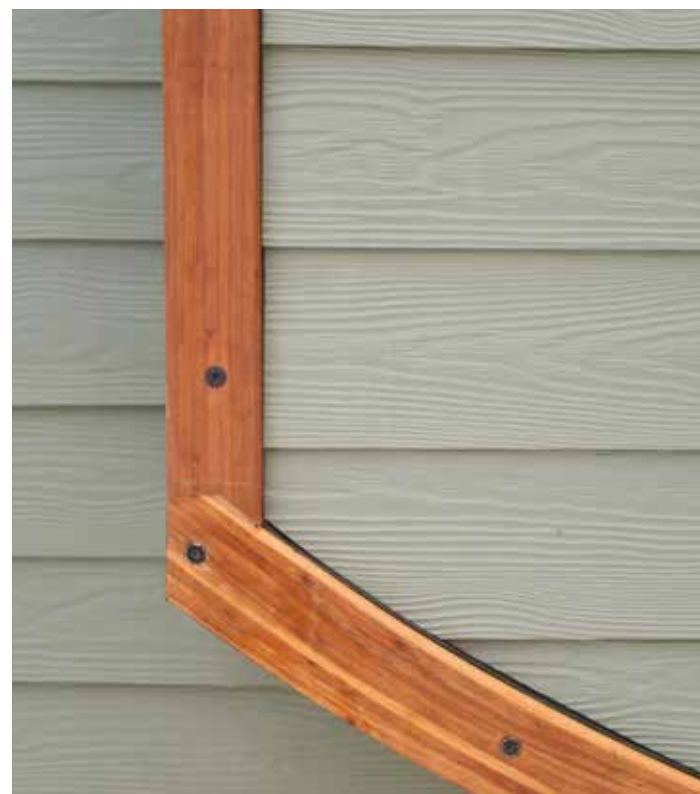
Built to last. Fiber cement siding is extremely durable, fireproof, and resistant to insects and Mother Nature.
