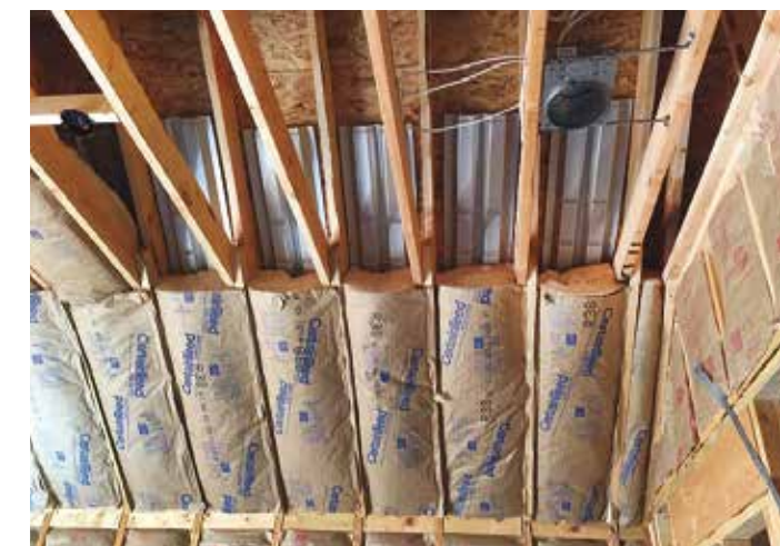
Vented Roof Slope Assembly
