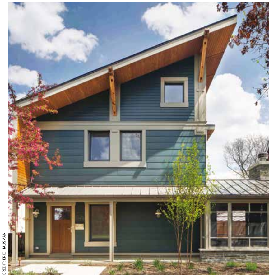
Green inside and out. Right-Sized Passive Home in Oak Park, Ill., was named Single-Family Project winner thanks in part to an interior with nontoxic, no-added formaldehyde, water-borne finishes, and a dedicated energy use monitoring system.
