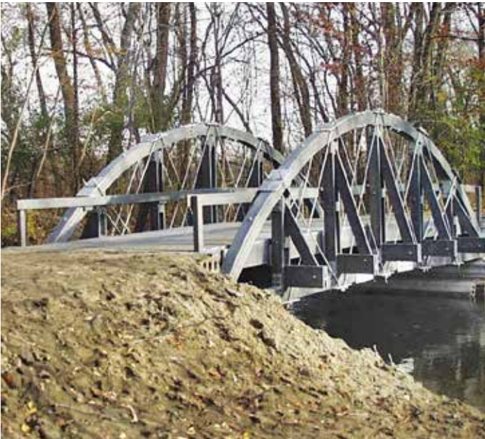
By the book. With careful engineering, plastic lumber has been shown to be feasible even for projects with higher load requirements.
