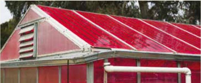
Surprise growth. Plants germinated in a smart greenhouse under translucent solar panels fared as well or better than those cultivated in conventional greenhouses.
