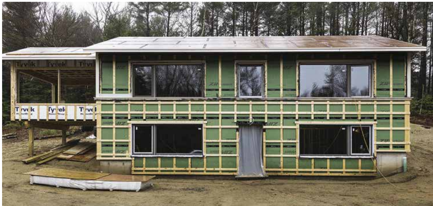
Staying power. ZIP System R-sheathing and polyisocyanurate continuous foam exterior insulation will help make this Westhampton, Mass., custom home energy efficient and able to withstand brutal New England winter weather.
