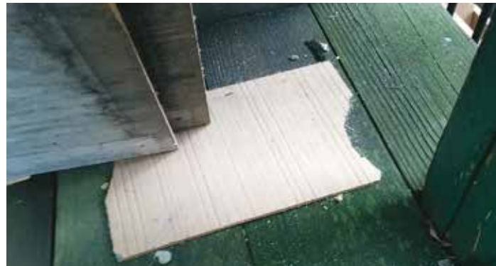
Red flag. Piles of asbestos-based shingles left exposed like this are a sure sign to OSHA that materials have been removed improperly. Only a licensed asbestos mitigator can remove large areas of material, particularly on multi-family homes.
