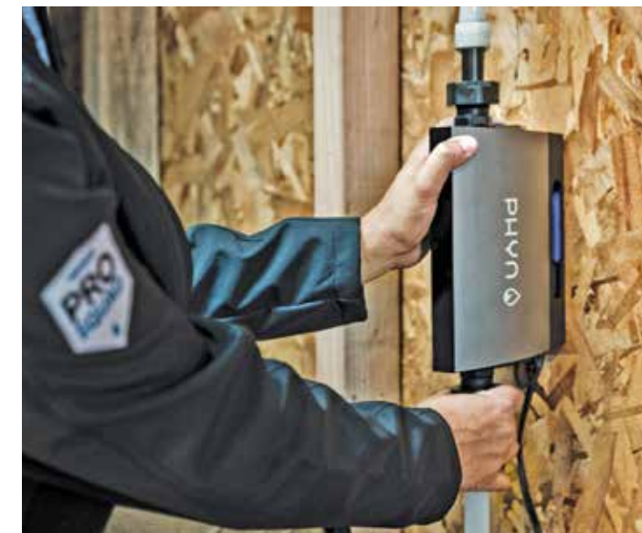
Water watch. Leak detectors, such as Phyn , demonstrate the potential for passive monitoring without video surveillance.
