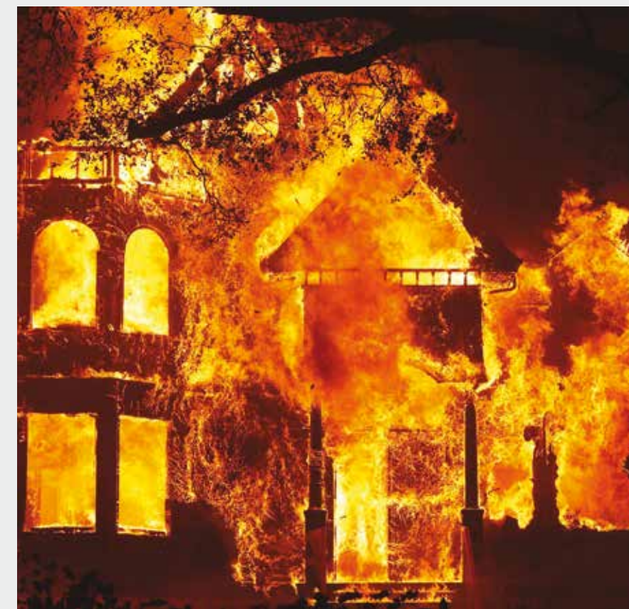
Burned out. The historic Glass Mountain Inn in St. Helena, California, was among the 1,555 homes, businesses and other structures destroyed during the 67,500-acre Glass Fire last fall.
