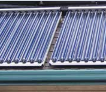
Sun Catcher. Flat plate and evacuated tube collectors are two technologies commonly used to capture solar energy for water heating.
