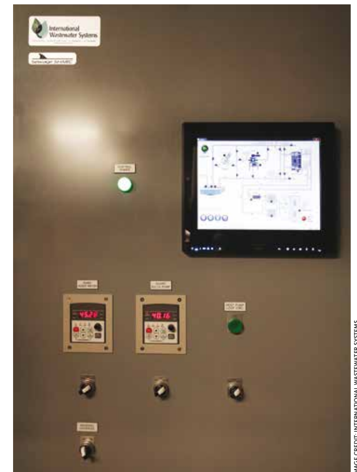
Ground Control. DDC system controls include a touch screen interface, data logging and remote monitoring capability.
