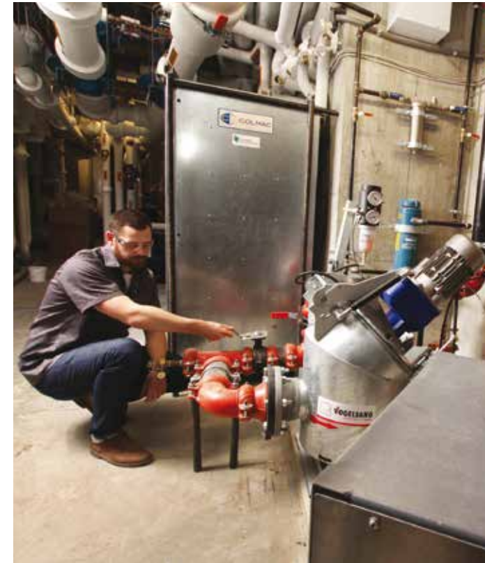
Heat Source. The Sewage SHARC from International Wastewater Systems processes raw sewage in preparation for recovering its heat energy. The system is fully sealed and odor-free.
