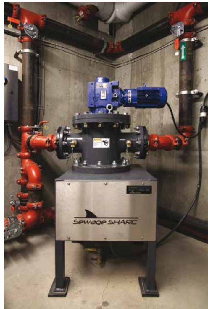
Components. The SHARC system includes the Sewage SHARC filter and heat exchanger, along with DDC controls. An in-line sewage macerator is optional.
