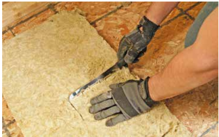
Natural materials. Roxul manufacturers stone wool insulation, which is made of of Basalt rock, a volcanic rock, and recycled slag, a by-product of the steel and copper industry.
