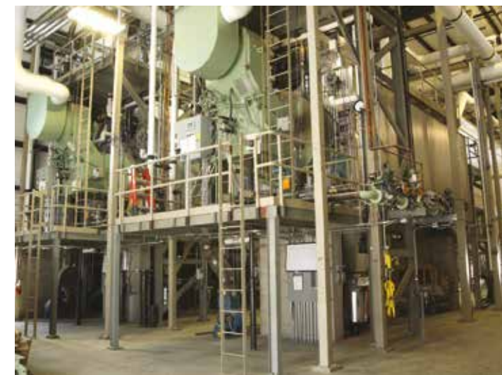
Sustainable investments. Andersen's $20 million energy plant injects sawdust into a boiler to create steam, which powers manufacturing equipment.
