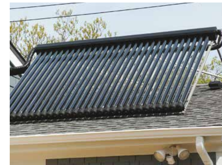
Solar water heating. The system includes two 30-tube evacuated tube panels and a 120-gallon storage tank with electric backup.
