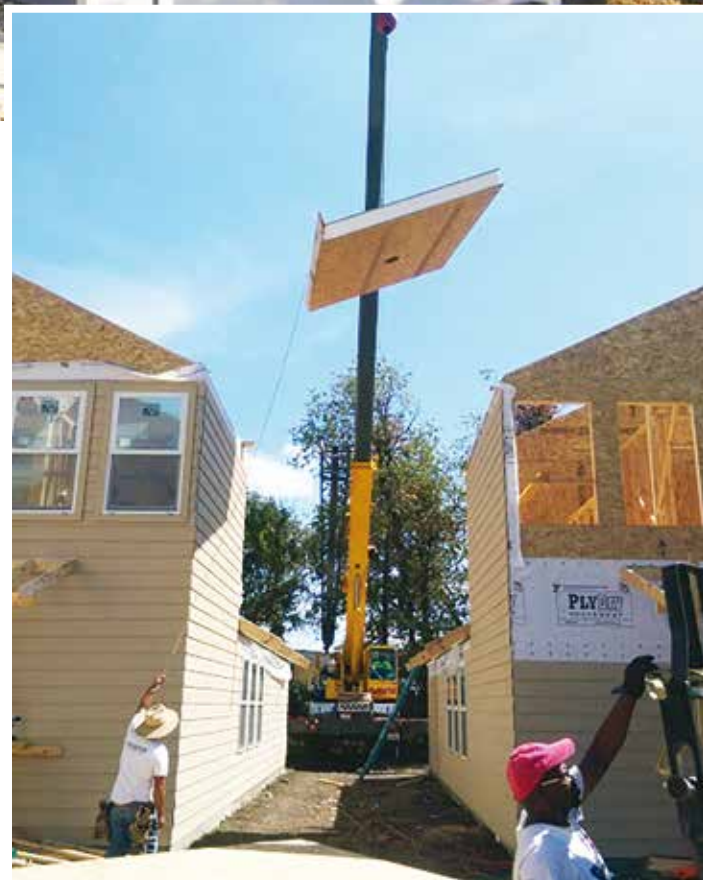
SIP construction. The SIP thermal blanket uses 8.25-inch-thick roof panels placed on the SIP walls.
