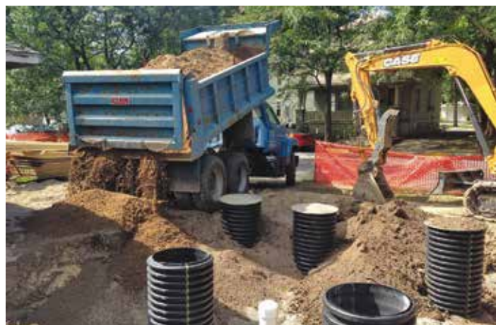
Rainwater. An underground rainwater collection system at the ReNEWW House in Indiana has a carrying capacity of 3,000 gallons.
