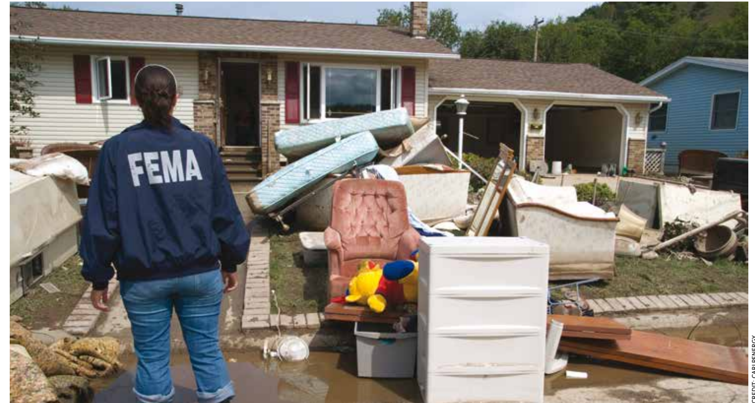
After the storm. Removing all moveable items quickly can save some household items after a flood, but carpets and drywall have to go.
