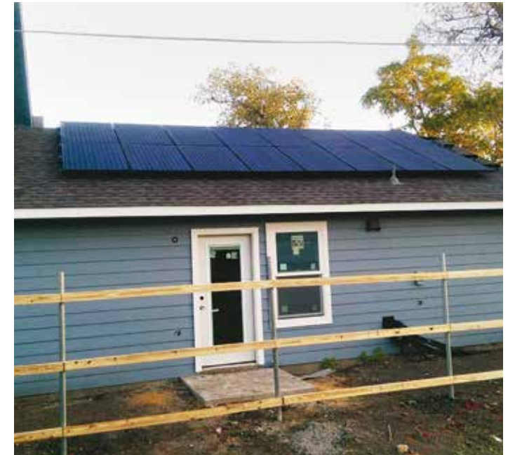
Saving with solar. The home includes 3.5 kW of solar electric panels that provide $1,905 in annual energy savings.
