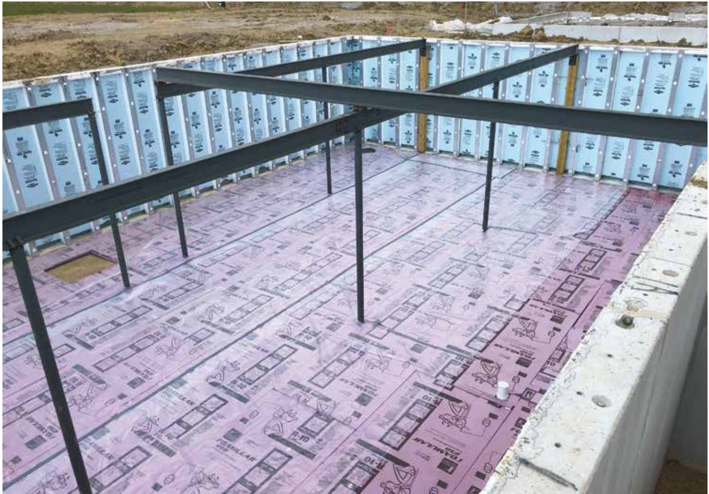
No thermal breaks. Exterior rigid insulation keeps below-grade steel framing encapsulated within the envelope. COURTESY OF GREENTECH CONSTRUCTION
