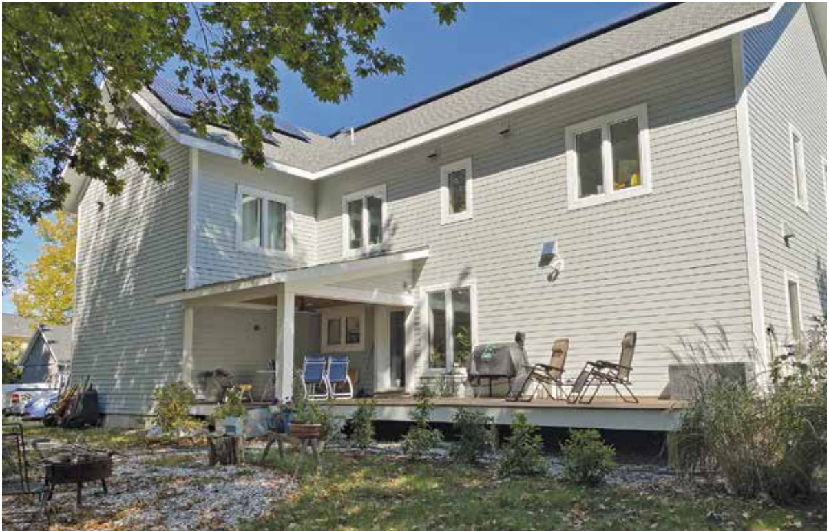
Outer limits. Zero-VOC paints, triple-pane windows and a solar array offer better control of the amount of energy used or lost during the day. CREDIT: WILLIAM FREEMAN
