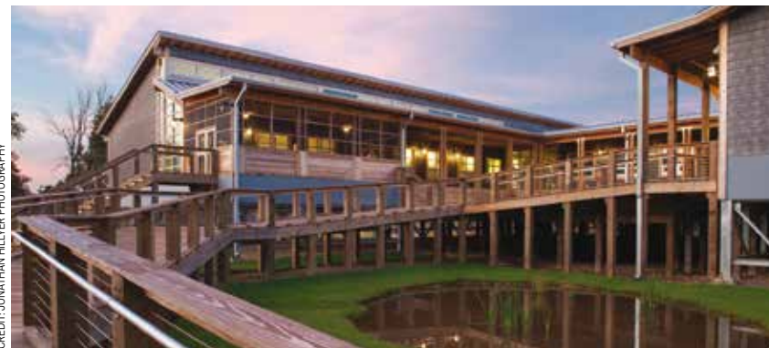
Flow on the go. Grand Bay Discovery Center's 12-foot-high trusses allow flood waters to move below unimpeded, reducing impact on the natural hydrology.
