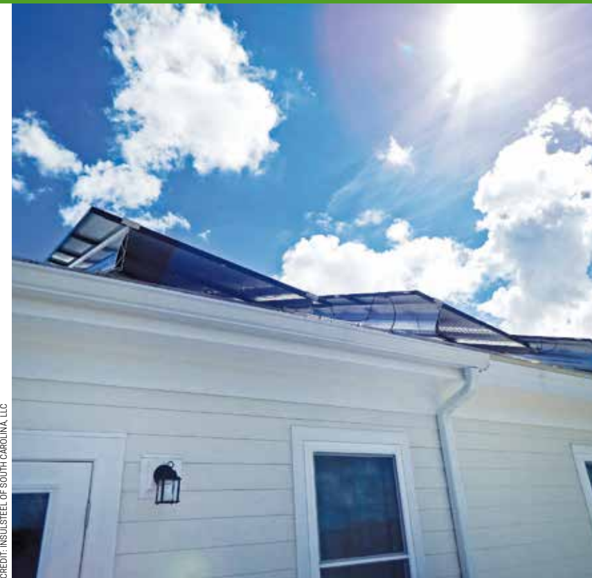
Let the sun shine. Solar panels are installed at the optimal angle for gathering light at this location. They have already survived a tornado without damage. The home also has two solar water heating panels.
