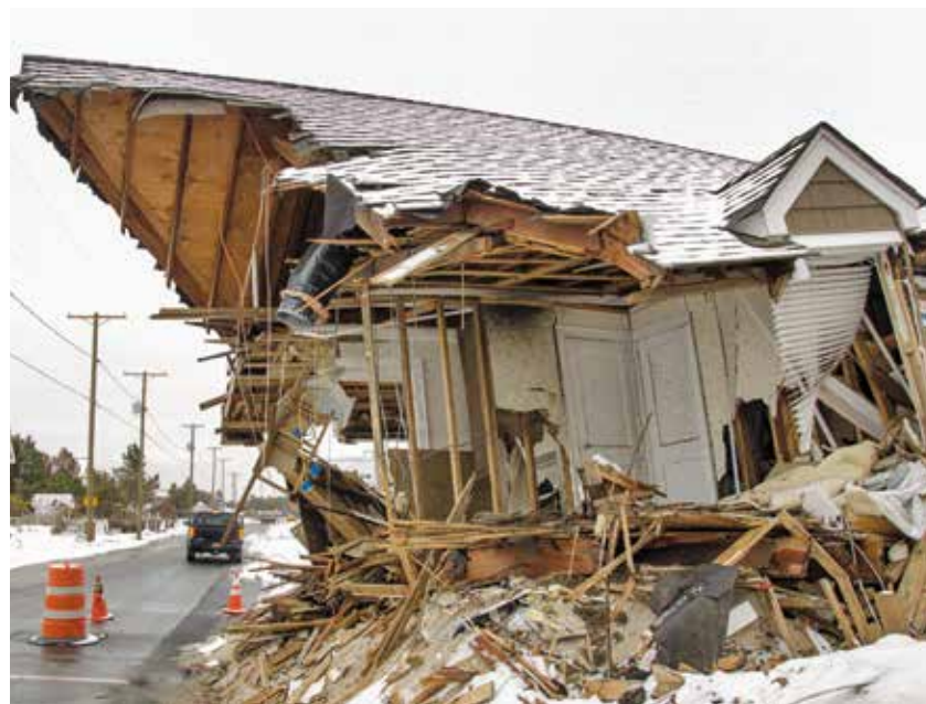
Age matters. Older building materials and systems perform much more poorly in high wind than new products built to better codes.
