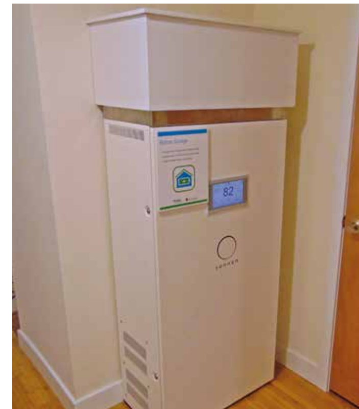
Saved for a rainy day. Each modular home's solar array charges up a sonnenBatterie smart energy storage system, in case the local grid goes down.
