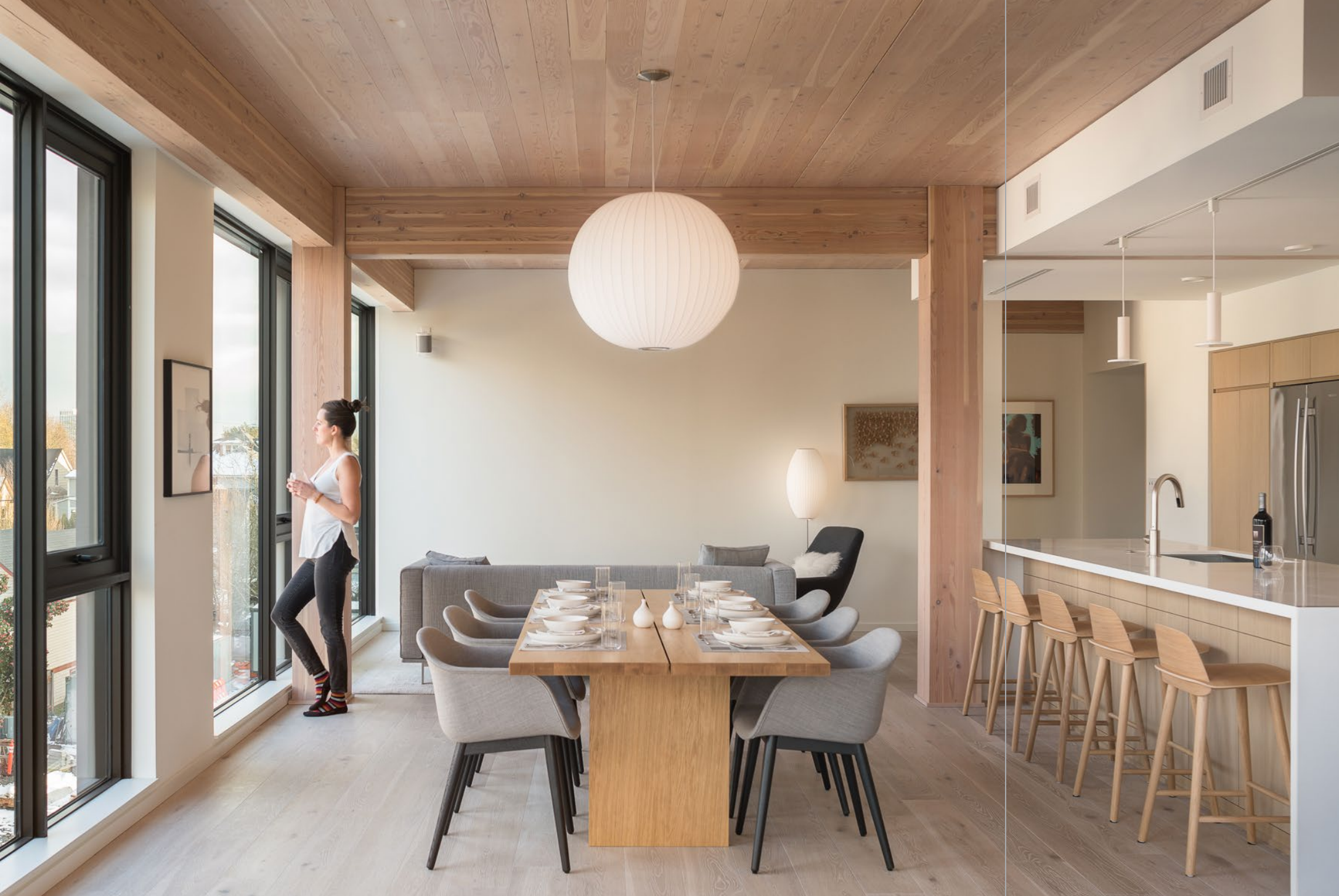
Carbon 12 shows off the beauty of wood with its exposed Douglas Fir panels doubling as finished ceilings.
