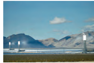
Space Age Reality. The Ivanpah Solar Power Plant in San Bernardino County, Calif., collects sunlight and focuses it on tall towers filled with liquid salt.
