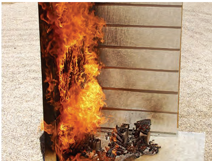
Siding Test. A burning brand applied to a test wall assembly at UC Davis set alight the composite wood siding (left side), but the fiber-cement-covered wall did not ignite.
