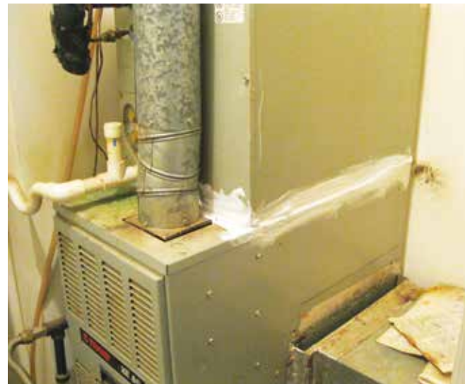
By Hand. Mastic was used to hand seal air handlers from the outside.
