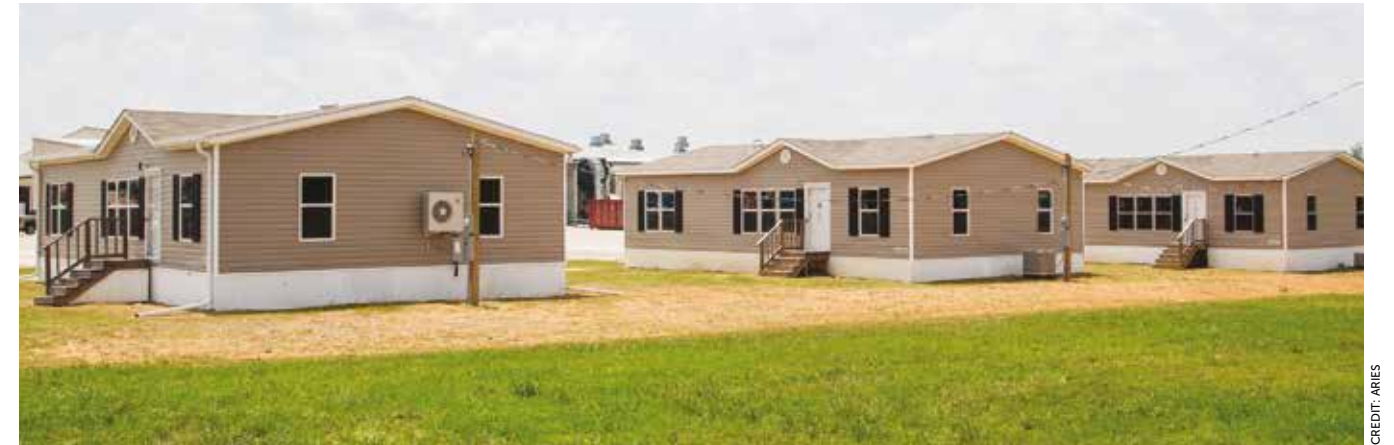
Side by Side. The dense-pack roof insulation technique is being tested in a side-by-side comparison with two other manufactured homes—one built to ENERGY STAR standards; the other built to the HUD code.
