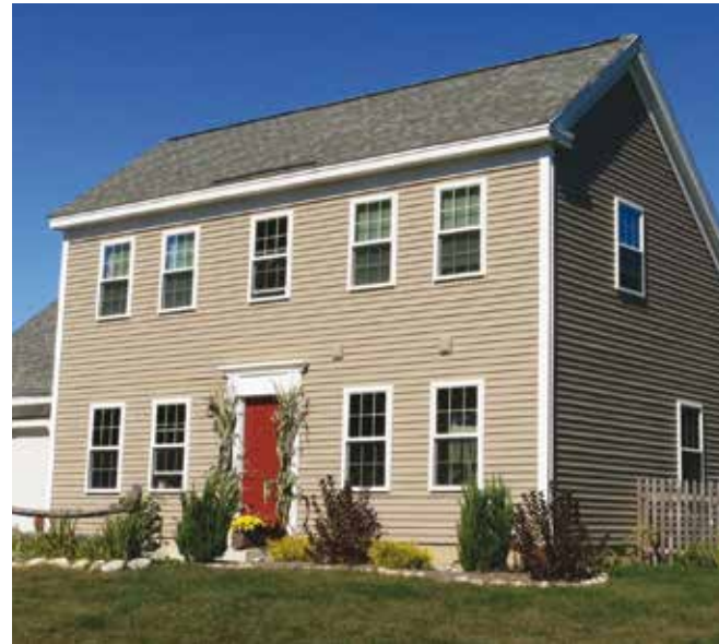
Transferred Savings. For a standard-size house, Transformations, Inc. saves $5,500 by using a simplified MSHP system and spends $15,000 on enclosure upgrades.
