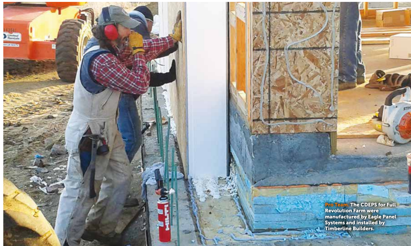
Superior Envelope. A CDEPS curtain wall installed against the framing adds insulation and eliminates thermal bridging.
