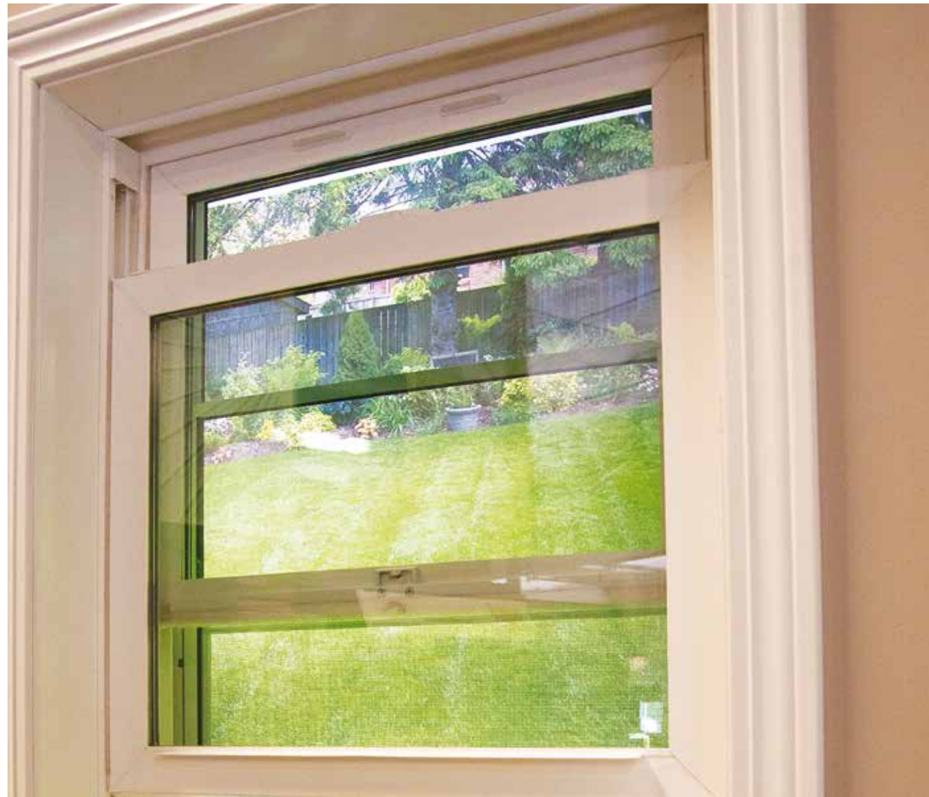
Inside Job. Storm windows, such as the interior unit shown here, can be custom ordered from window distributors and some big box retailers. Some common sizes are available off the shelf.
