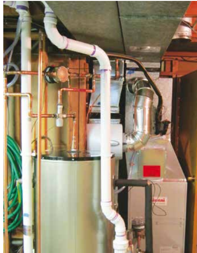
Upgrade. The retrofitted combi systems typically operated in the condensing mode and provided acceptable, and in some cases, improved occupant comfort.
