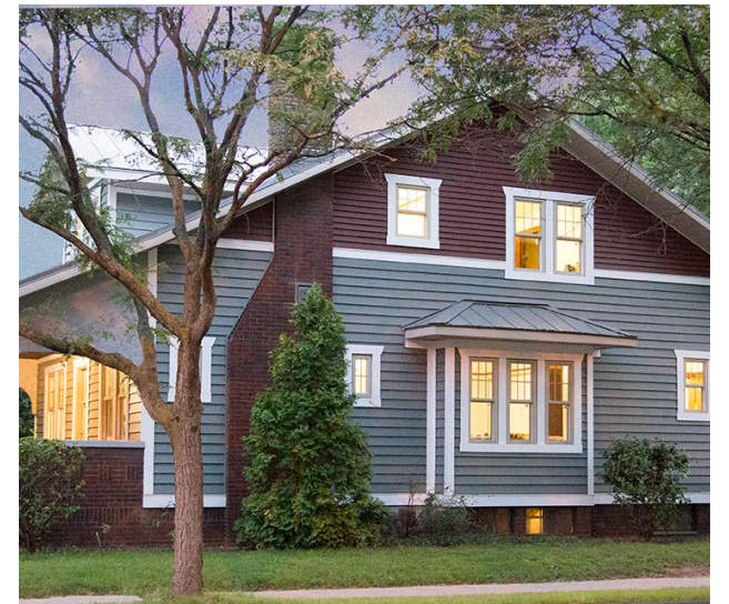
The ReNEWW house siding incorporates a polystyrene foam insulation backing that wraps the home’s exterior envelope with a continuous blanket of insulation up to 1.25 inches thick, helping to minimize air leakage and break any thermal bridges. The siding is also manufactured with 50 percent recycled materials. Ply Gem Cellular PVC Trim, a low-maintenance alternative to traditional wood trim that is designed to work well with nearly any siding type, is utilized throughout.
