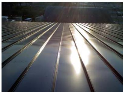
With the solar re-roof, the old roof is covered with a long life, weathertight roof and solar heated air is delivered to the building to supply: direct space heating of the gym, outdoor air preheating for the gym, and domestic hot water preheating.
